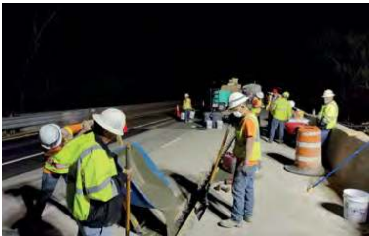
↑ Construction with UHPC Concrete; the United States
