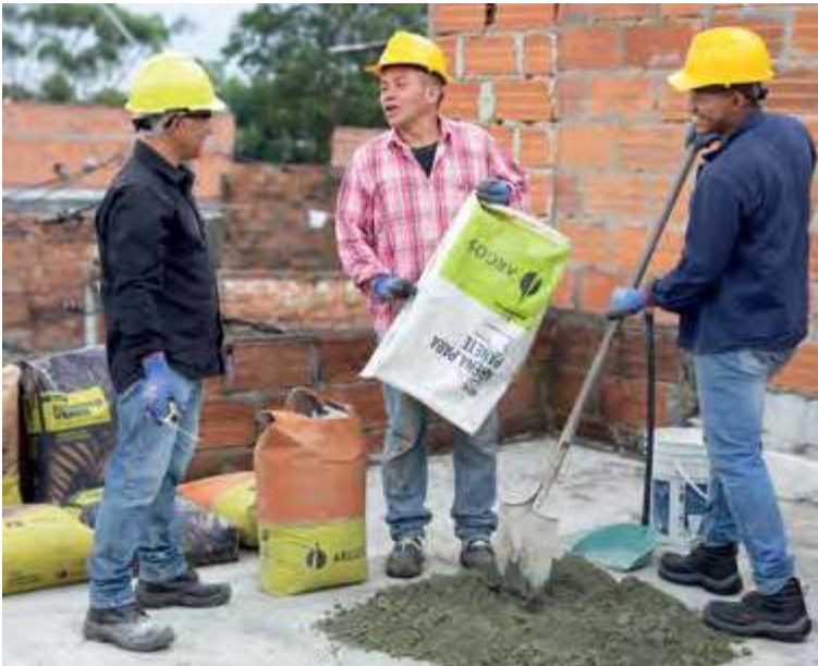
Construction workers; Colombia
