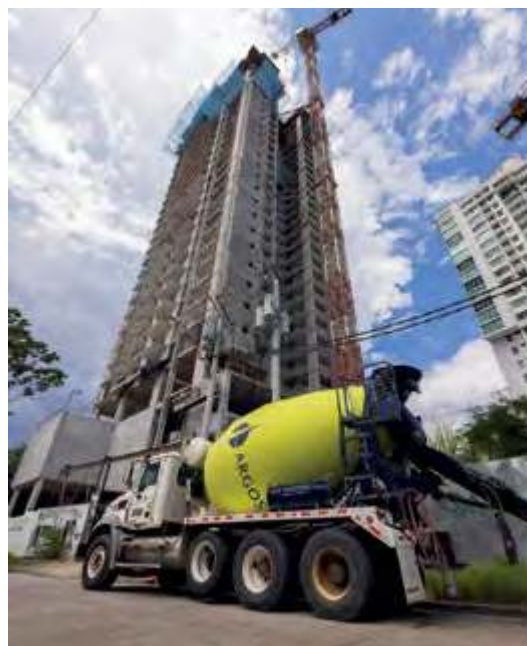
↑ A mixer truck on site; Panama
