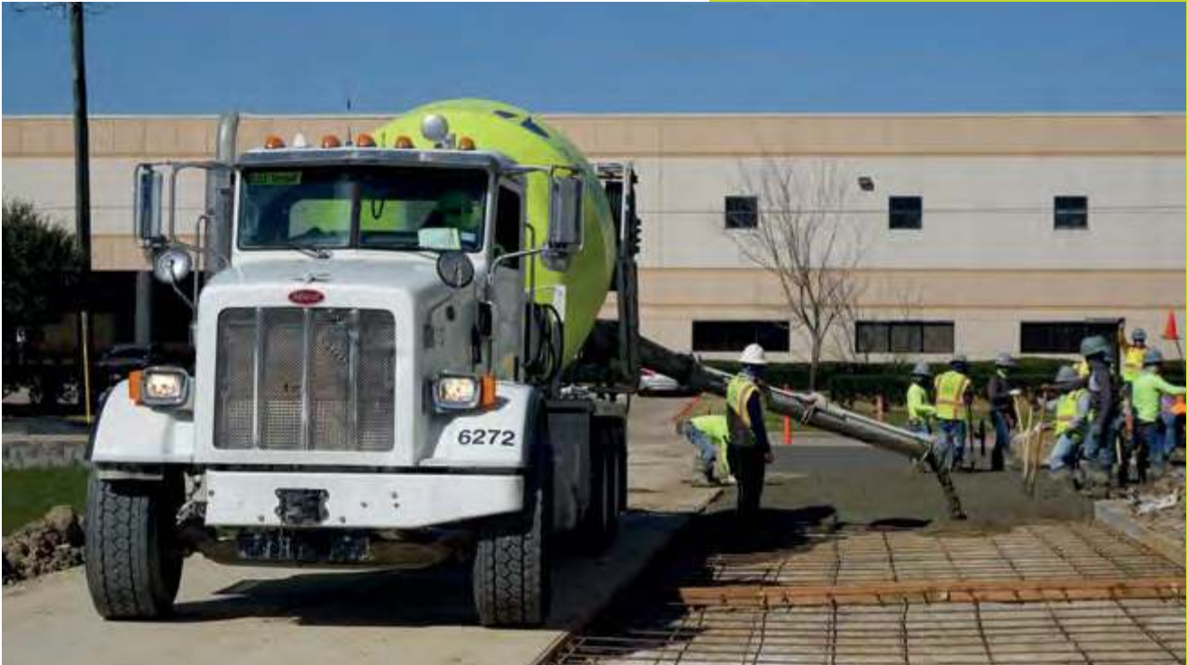
↑ Concrete pouring in Houston, the United States
