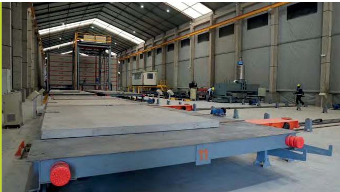
↑ The Concrete Modular Plant, in Cajicá, Colombia
