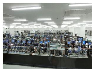
Clean room with latest air-conditioning system
