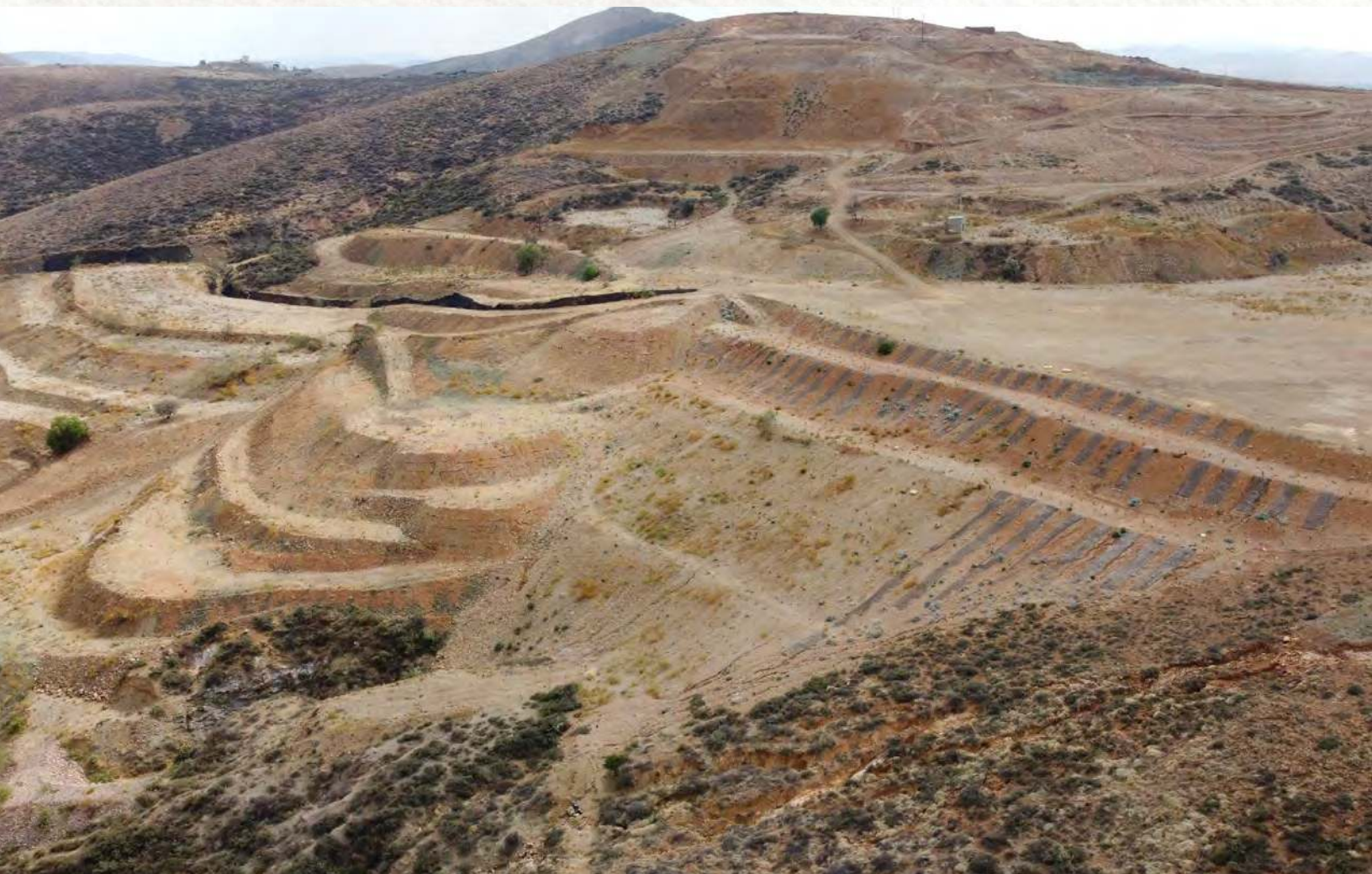
Cozamin – Chiripa TSF Reclamation
