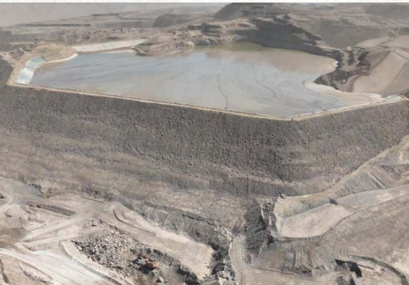
Mantos Blancos – Pit Phase 8, Stage 4 Construction
