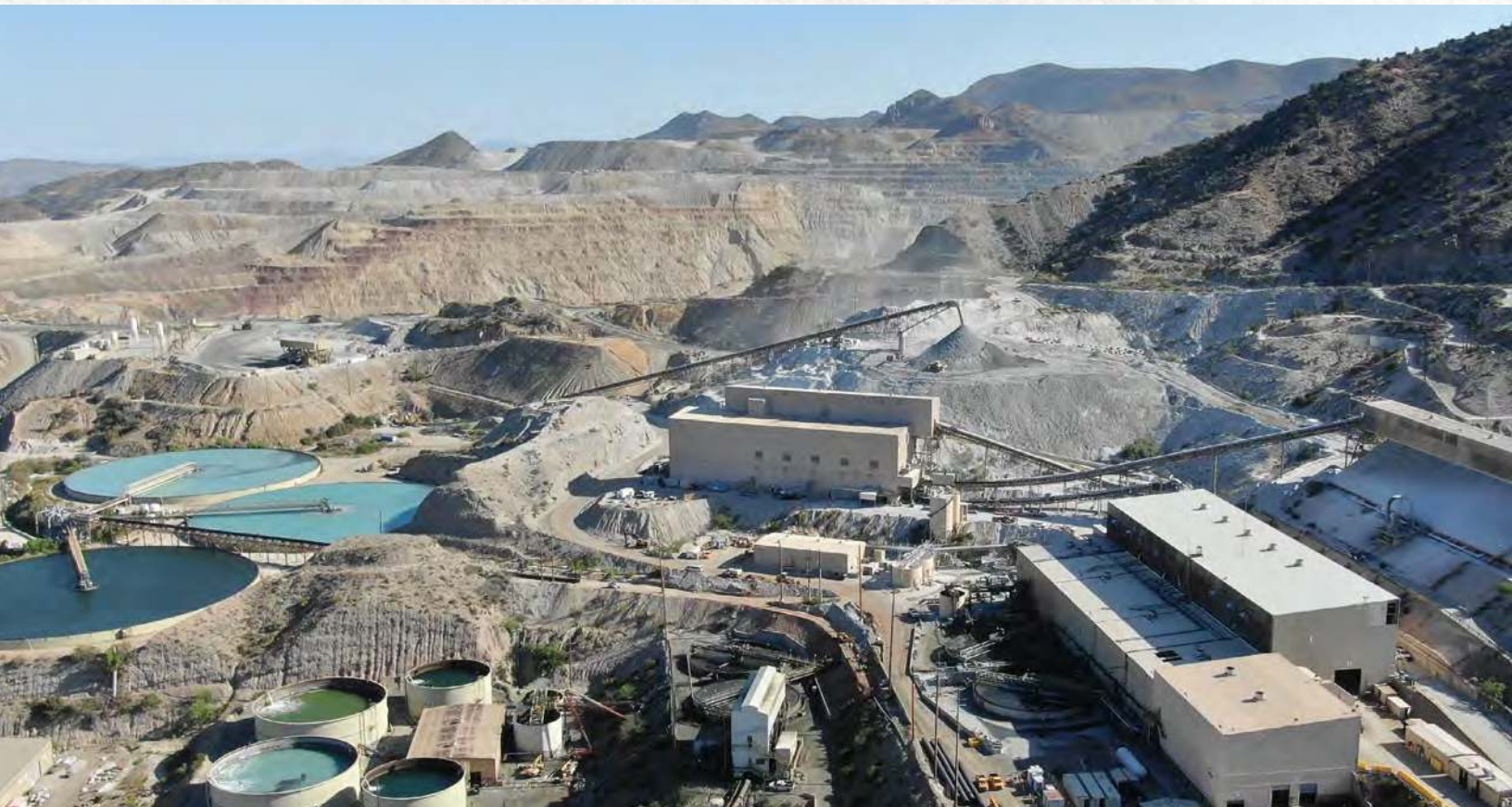
Pinto Valley – General View of Processing Plants
