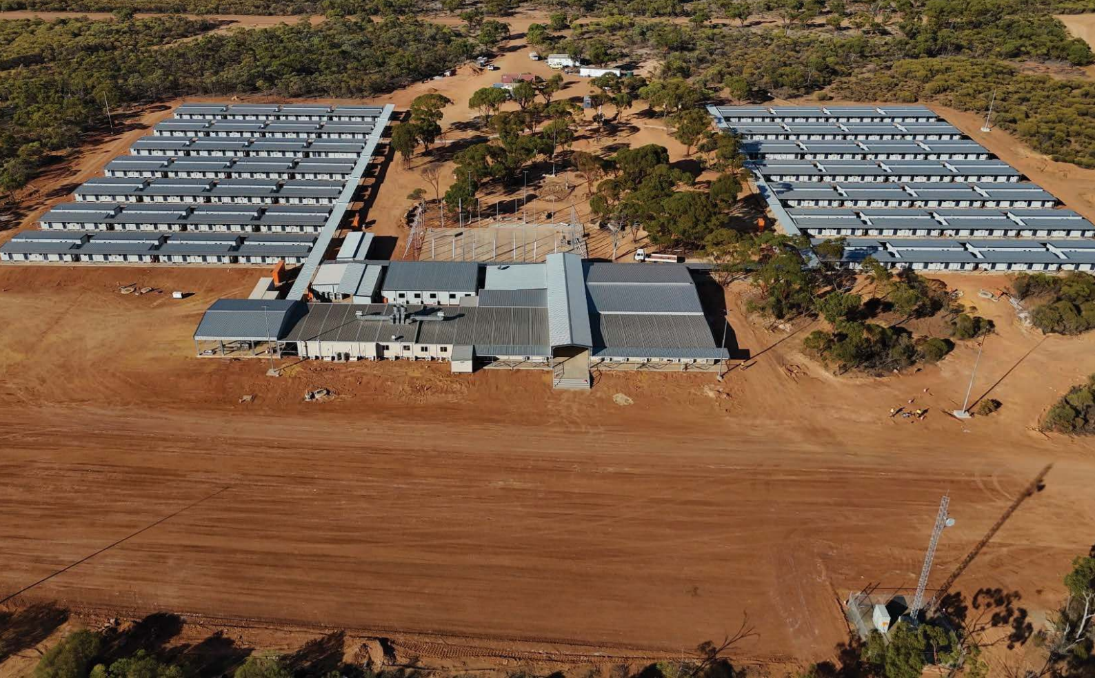
Mt Gibson Gold project – accommodation village installation
