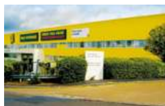
Staples Corner, March 2001
