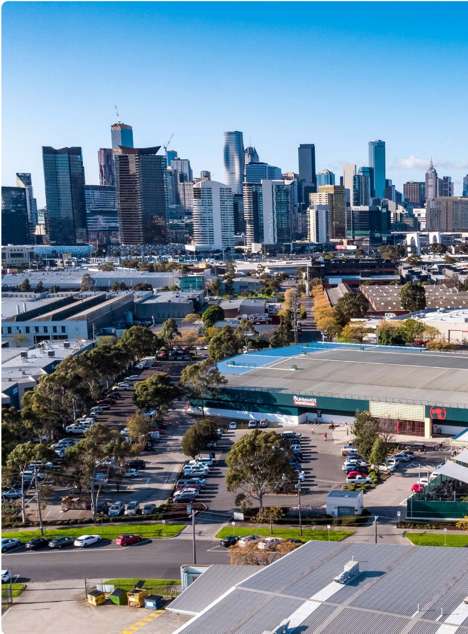
BUNNINGS WAREHOUSE PORT MELBOURNE, VIC
