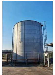
100,000L rainwater tank at the Cornubia Service Centre.
