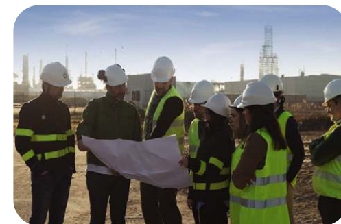
Image: Construction has begun on the green hydrogen project at our Castellón refinery, Spain
