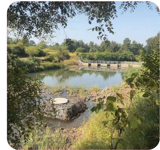
Image: Check dam and recharge well in Silvassa, India
