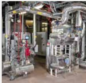
Environmentally friendly cooling system and a high-temperature heat pump at the Ennstal dairy farm in Austria, installed by Equans
