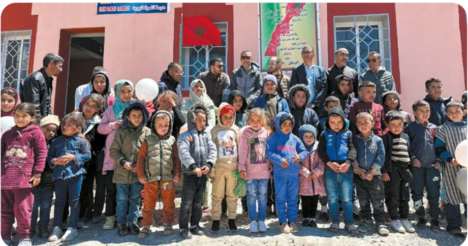
MOROCCO – Reconstruction of a school and lavatories in Talmoute Tabourite, Morocco, by the non-profit "Enfants du Désert", with the support of the Bouygues Construction Foundation.
