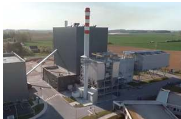
supplying steam to the Bonduelle plant in Estrées-Mons (France).
