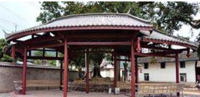
Beautiful Village Construction in Zhezhen Village
