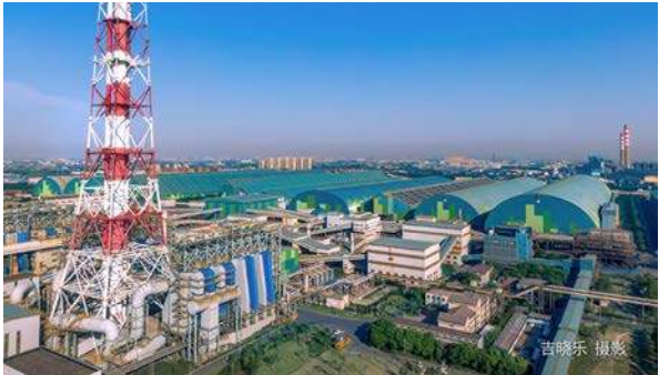
Enclosed Raw Material Storage Yards at Baoshan Base
