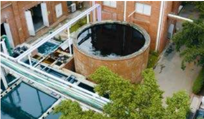
Bangladesh A water purification plant located at one of our suppliers.
