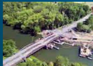
UK: Nuneham rail viaduct restoration, Network Rail.
