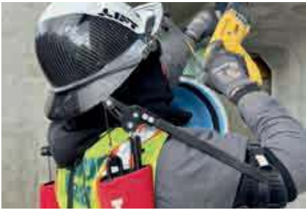
ABOVE Exoskeleton in use on the Harkers Island Bridge replacement project in North Carolina.
