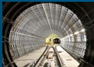
UK: London Underground Piccadilly line upgrade.
