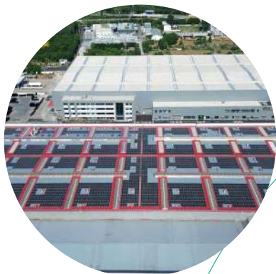
▲ Rooftop photovoltaic installation
