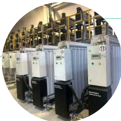
▲ Adsorption-type vacuum-assisted heating dryer
