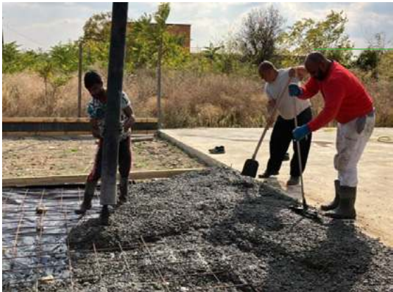
Floor slab of a private house
