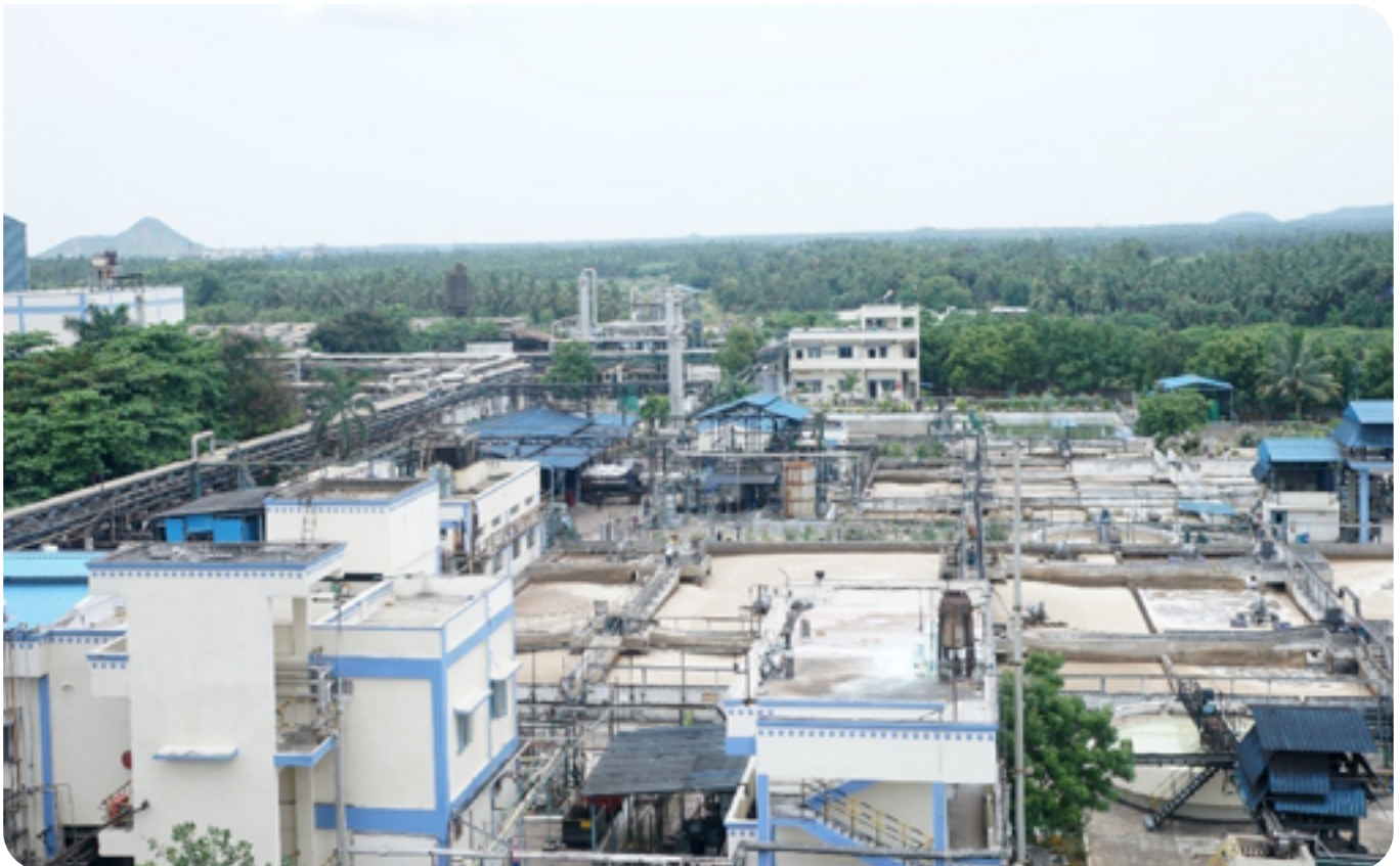
Effluent Treatment Plant
