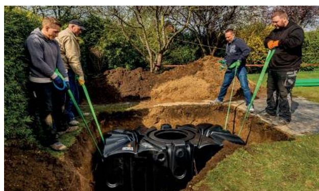
Installation of a Rainwater Harvesting Tank
