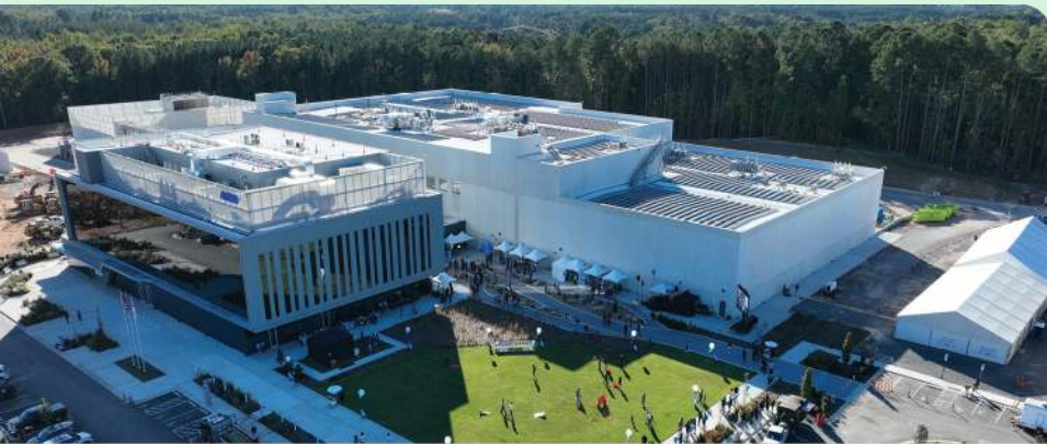
Amgen Ecovation™ principles guided the design and construction of our new state-of-the-art facility in North Carolina.
