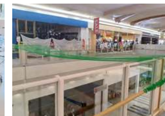
Safety net in case of ceiling collapse
