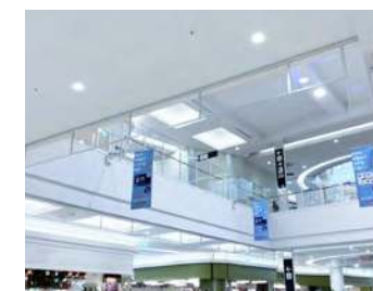
Smoke-proof hanging walls
