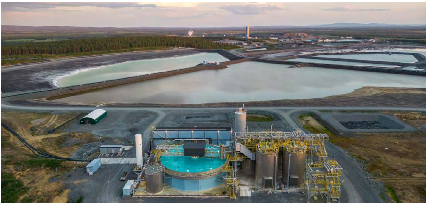
Water treatment plant at Kittilä (Lapland, Finland).
