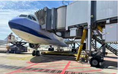
Replacing APU with GPU via Jet Bridge for Enhanced Efficiency and Emission Reduction
